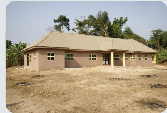
Isumpe Community Town Hall
