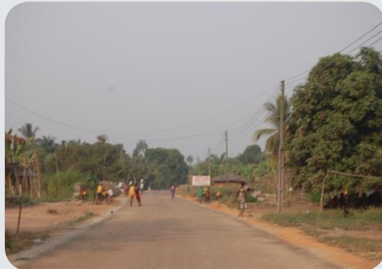
Obodugwa Internal Road Construction
