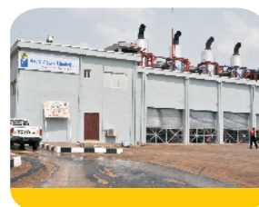
Commissioned 12.15MW Akute Power Plant
