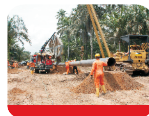
Achieved 90% completion of 128km Eastern gas pipeline
